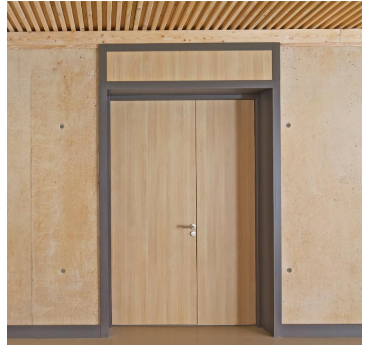
Final structural wall after demoulding and drying Maison des associations. Mil'lieux architects
